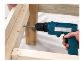
APPLY glue to the outside of the  $2\times4''s$  and then, using a power drill, SCREW the  $1\times8''$  to the  $2\times4''$ .
