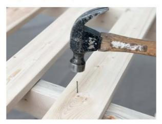
SECURE the bed slats by nailing them in place with finishing nails.
