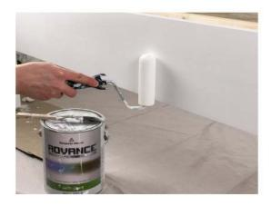
When your primer and caulking are all dry and your bed frame is sanded and wiped down, APPLY one to two coats of your topcoat paint.
